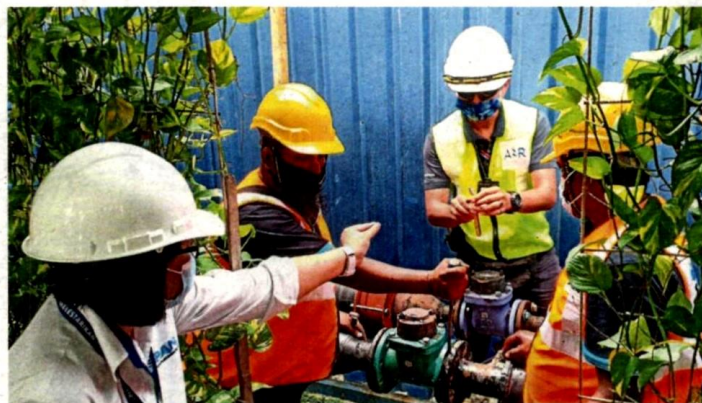
Loh (left) overseeing the work to dismantle the illegal pipe.
