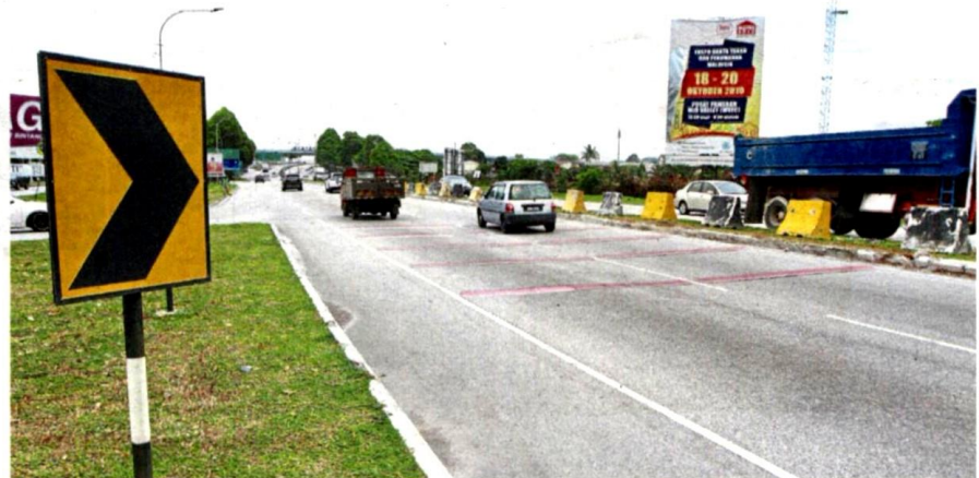
MPKJ has placed concrete barriers on the divider after a fatal accident took place along Persiaran Saujana Impian. — Photos: LOW LAY PHON/The Star
